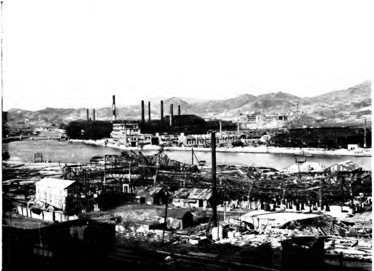
Photo No. 4. NAGASAKI. A general view showing some of the industrial buildings. That in the foreground was a gutted woodworking plant, just over a mile from the centre of damage, which was beyond the group of chimneys of the Mitsubishi Steel Works, seen in the middle distance. See paragraph 15.
